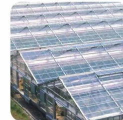
• Installation of PC board and endurance board.
