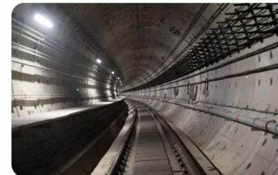
• Splicing of tunnel waterproof board.
