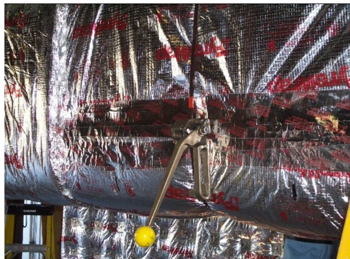
5. Fix material in place steel bands and/or pins where needed.
