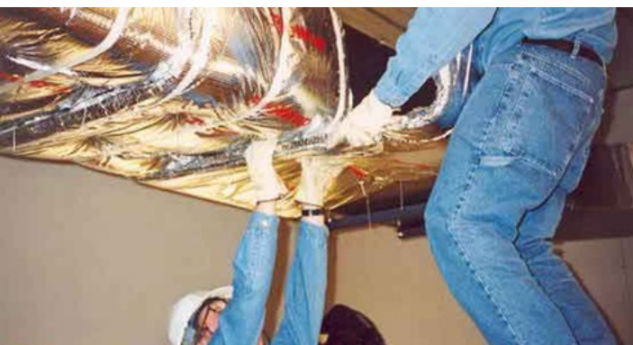
3. Telescopic overlap (most common method) - Wrap the blanket around the perimeter of the duct. Place the next piece of material with a 75mm (3") overlap of the adjacent material (circumferential joint) and 75mm (3") overlap where blanket meets itself (longitudinal joint).
